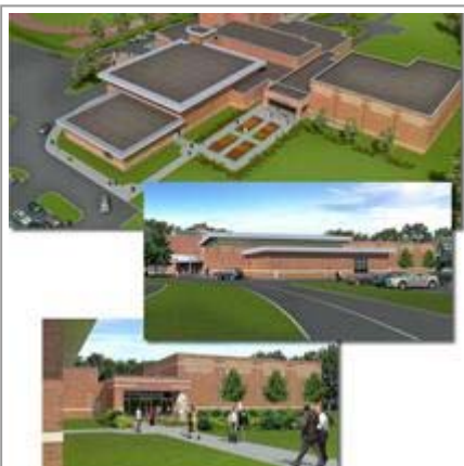
Ground breaking took place Monday for a $12 million expansion and improvement project at Notre Dame Academy in Park Hills. The work, expected to take five years, is being done by the Paul Hemmer Companies. (Courtesy Paul Hemmer Companies)
